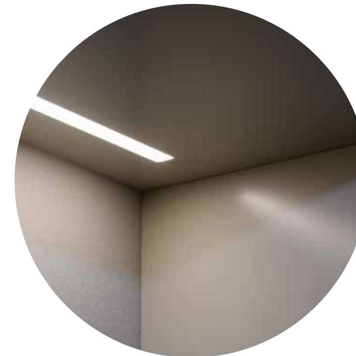
DETAIL LED STRIP IN MUURPLANK
